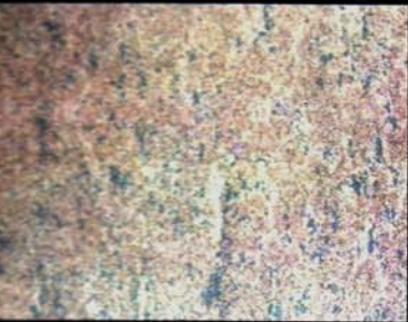
Condition A Blasted to Sa1
