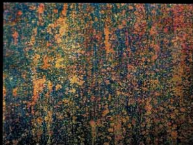
Condition B Blasted to Sa1
