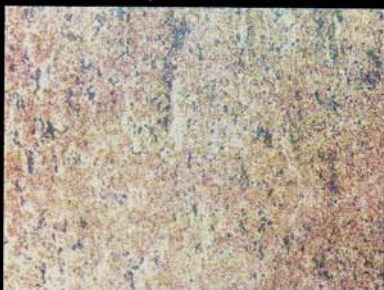
Condition B Blasted to Sa2
